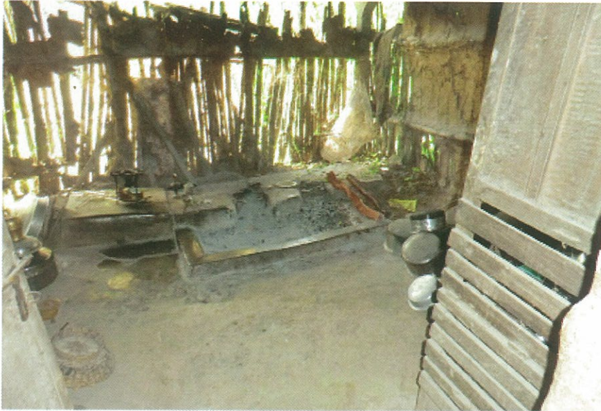
The abysmal condition of the inside of a hut
